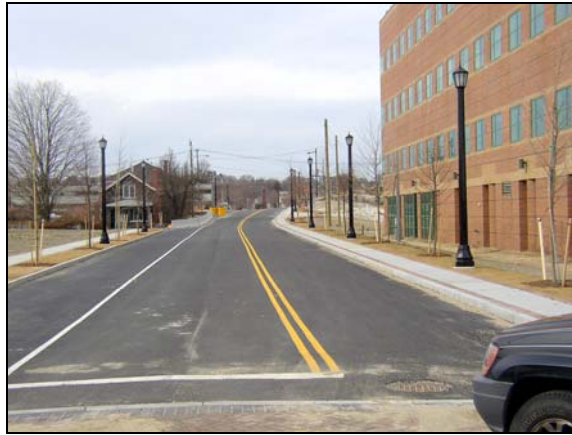
Looking west on the south side of Chelsea Street was the last occupied house at Fort Trumbull (since removed). Note how it blocked the sidewalk and road improvements.
